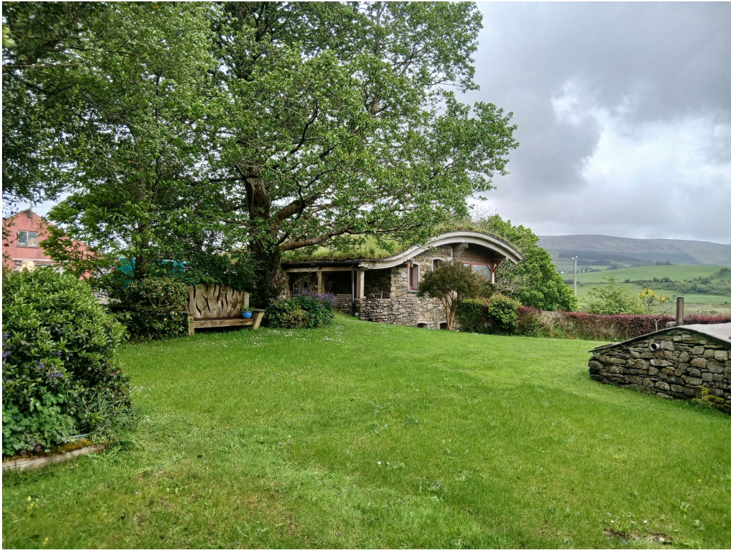
Photograph 2. The house at Maulikeeve. Self-designed and built with stone from the surrounding hillside, wood from recycled timber frame panels, and beams and posts from locally sourced trees. The curved green roof is designed to emulate the rolls and curves of the surrounding landscape. May 2026.
